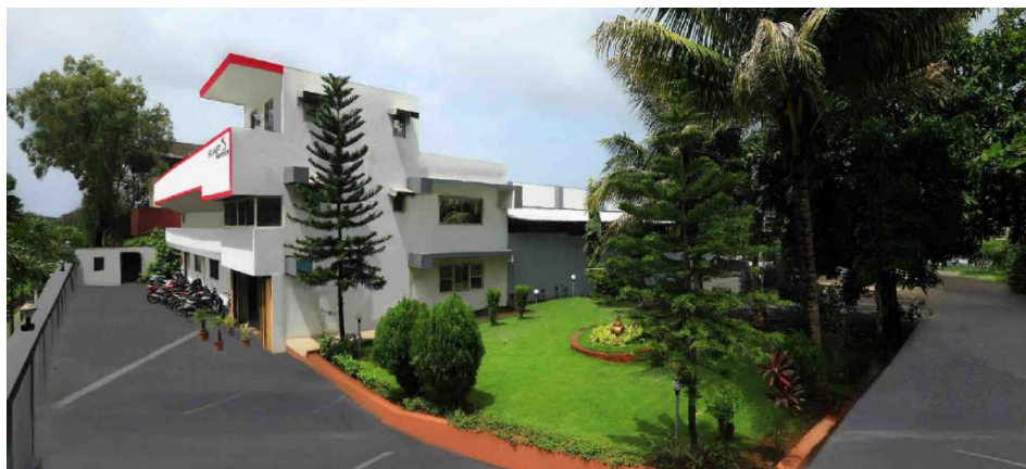
Side view of office premises
