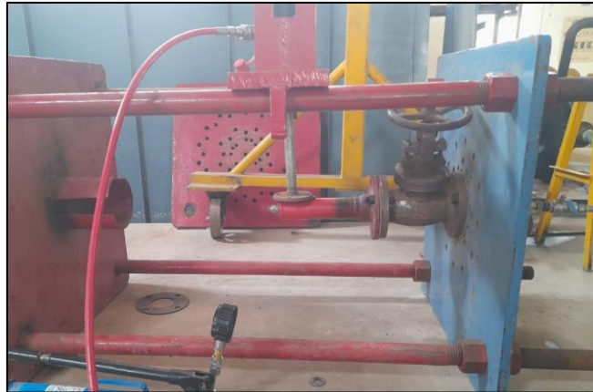
Figure 1: 65NB PN10 PIPE WRACKING SETUP
