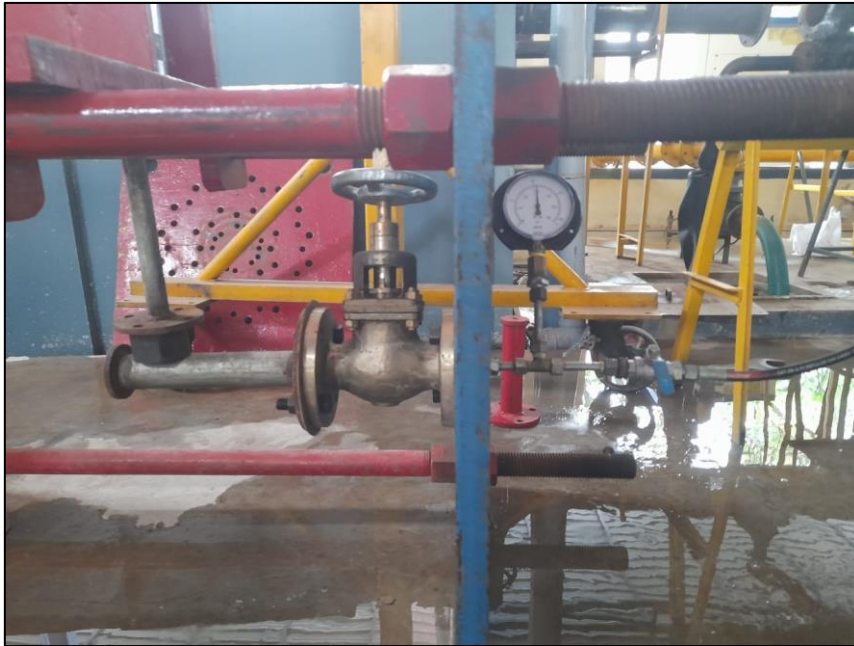
Figure 1: 50NB PN10 PIPE WRACKING SETUP
